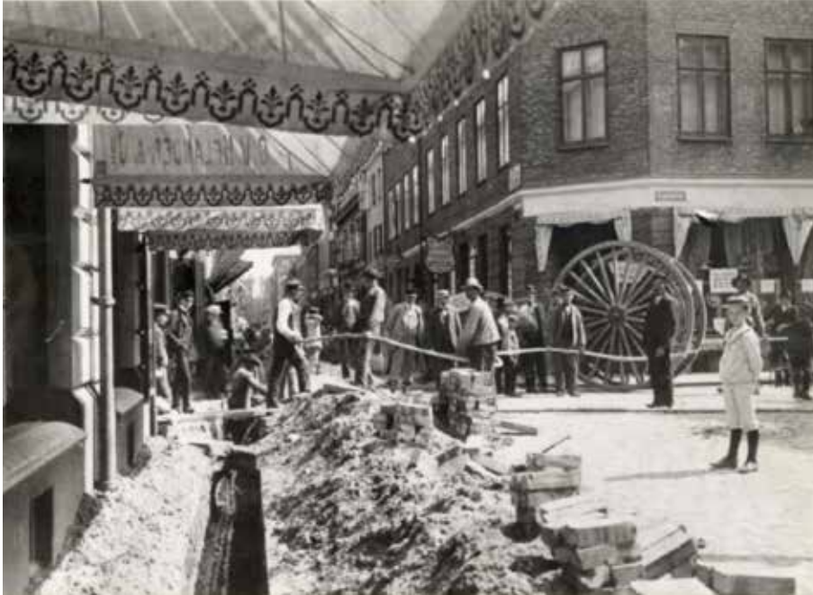
Wiring (1907–1908) at the corner of Kyrkogatan and Korsgatan, Göteborg.
